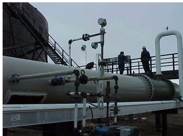
Slip stream (by pass) installation during commissioning
